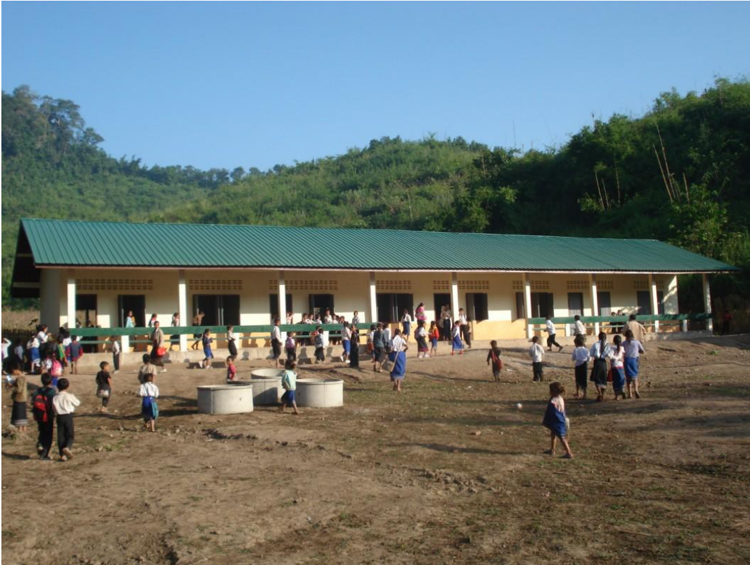
Overview of the new building
