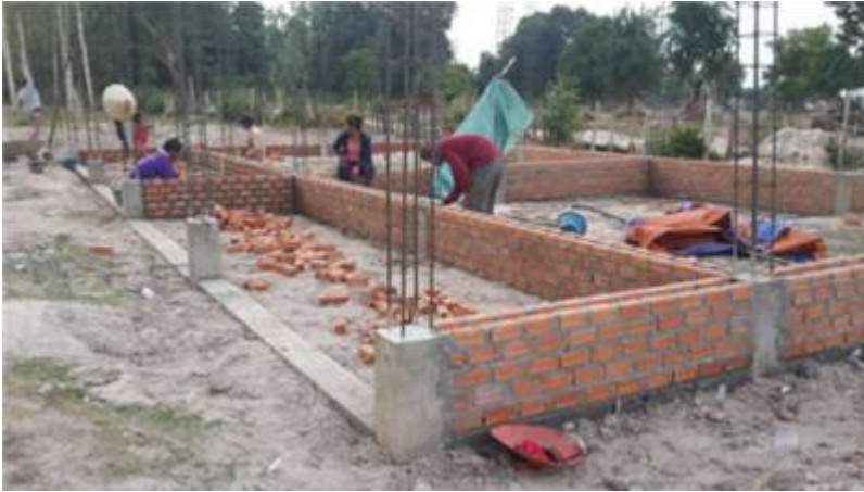
The foundation of the new building.
