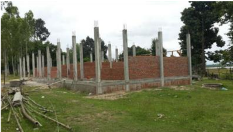
Front view of the new building in progress.
