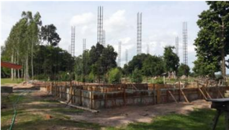
Construction of the ground floor.
