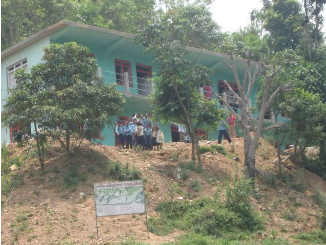
Newly constructed school building.
