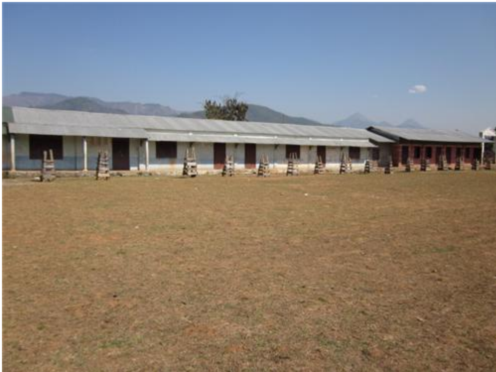
An outside view of some of the existing school buildings.
