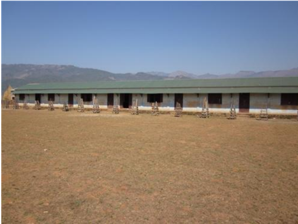
An outside view of one of the existing school buildings.
