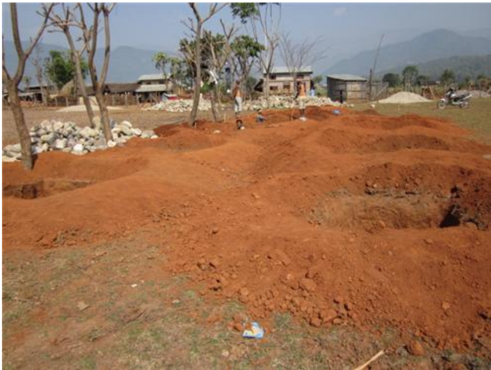
Excavation of trench.
