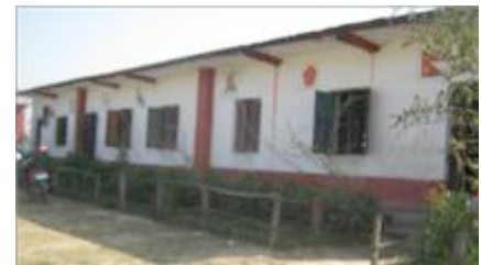
One of the existing school buildings that are in satisfactory condition.
