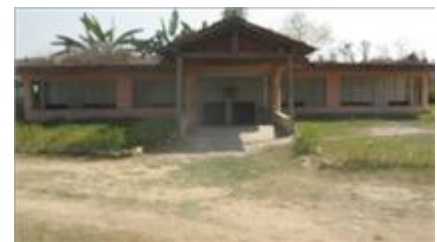
The main building of Shree Janjyoti Lower Secondary School.
