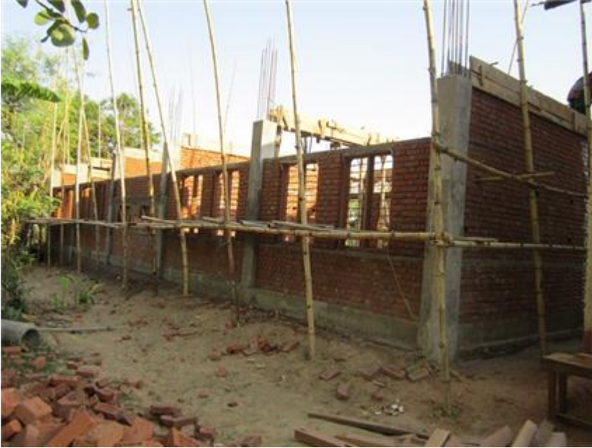
Ground floor construction work
