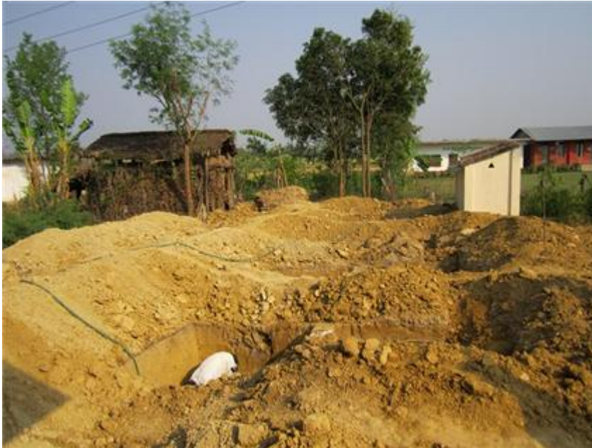
Excavation of the foundation
