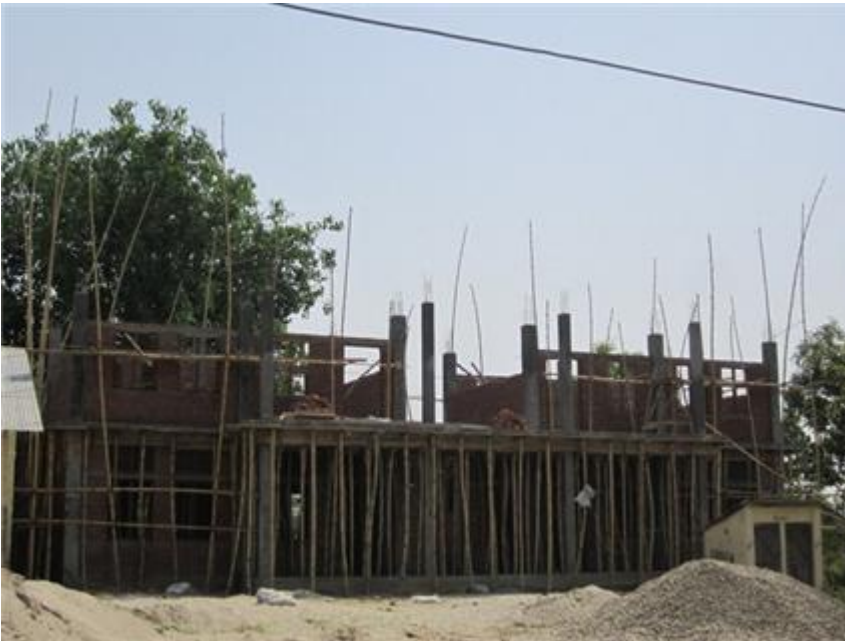
Progress of first floor construction work
